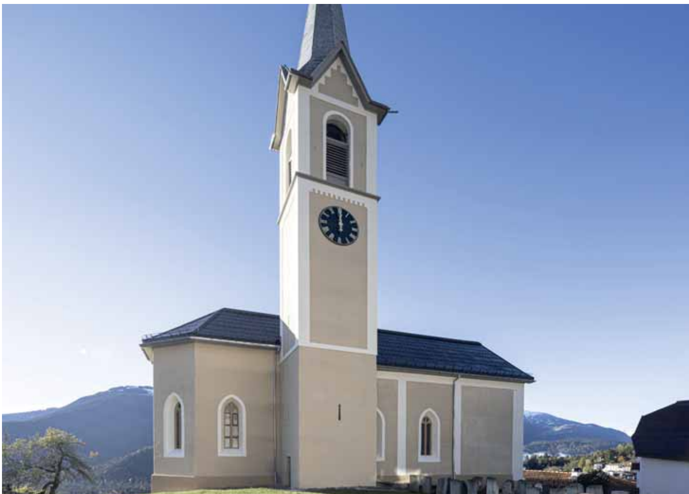
Fig. 1: The PV modules were not simply mounted on the main roof, but the roof itself was integrated into a PV building component in a complex process in accordance with Art. 642 Para. 2 of the Swiss Civil Code. This commitment to the medieval church deserves the Norman Foster Solar Award 2024.
